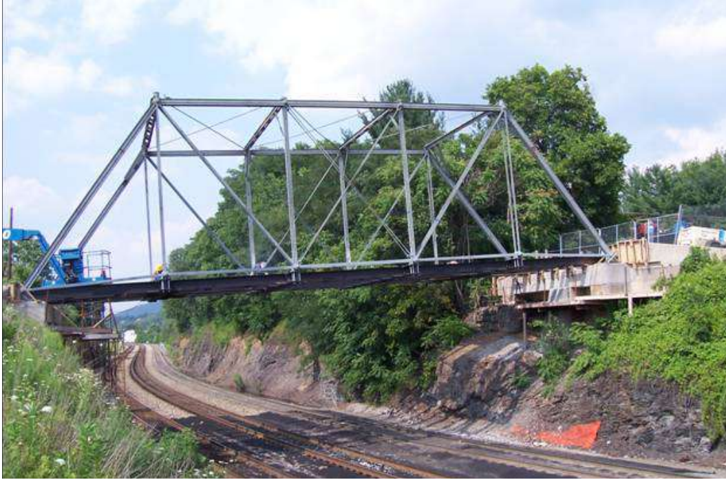
Figure 5.1 Hawthorne Street Bridge, Covington, Virginia
