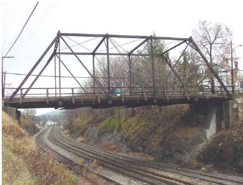
Figure 4.1 The Hawthorne St. Bridge in Covington, VA
