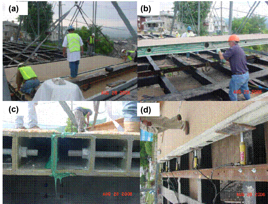
Figure 4.18 Field installation of the FRP bridge deck (a) Dry fit (b) Adhesive application (c) Seam curing (d) Jacking system
