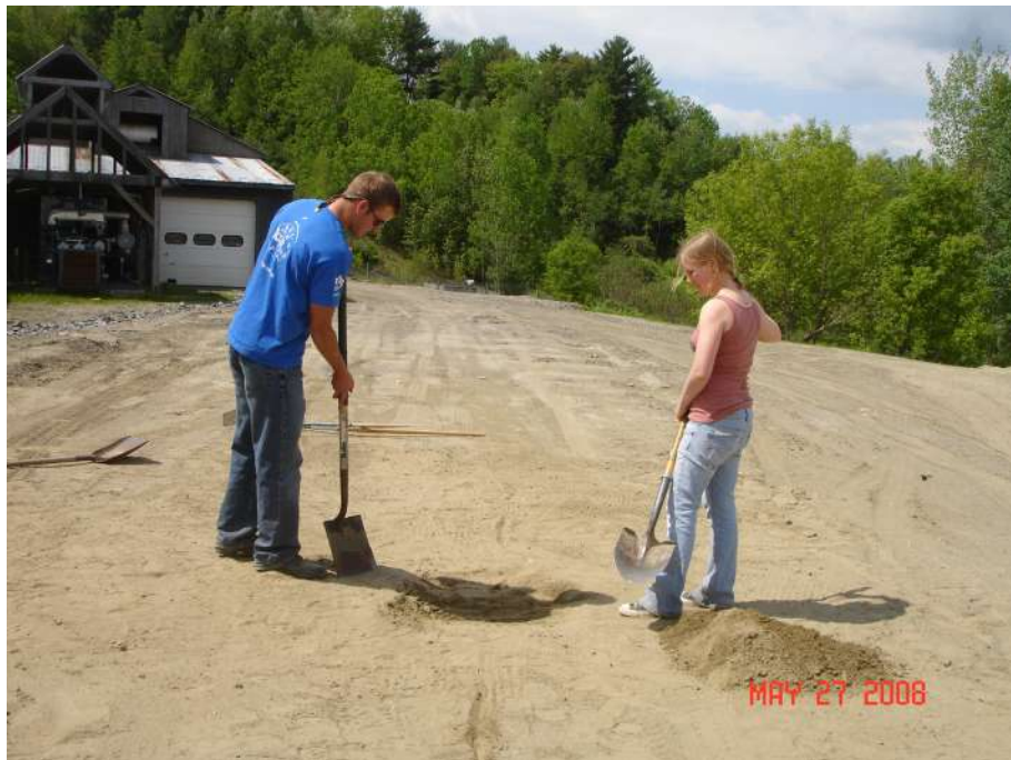
Figure C1. Test section, 27 May 2008.
